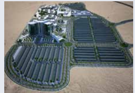
CIS thin-film modules with 10 MW capacity at the Saudi Aramco North Park Project (Saudi Arabia)
