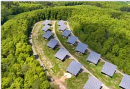
Radelstetten solar farm – 1.7 MW tracked PV plant on converted land
