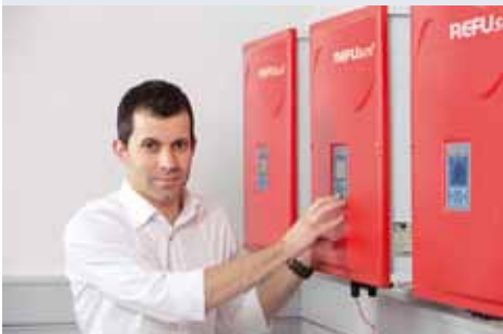
REFUsol training center in Metzingen
