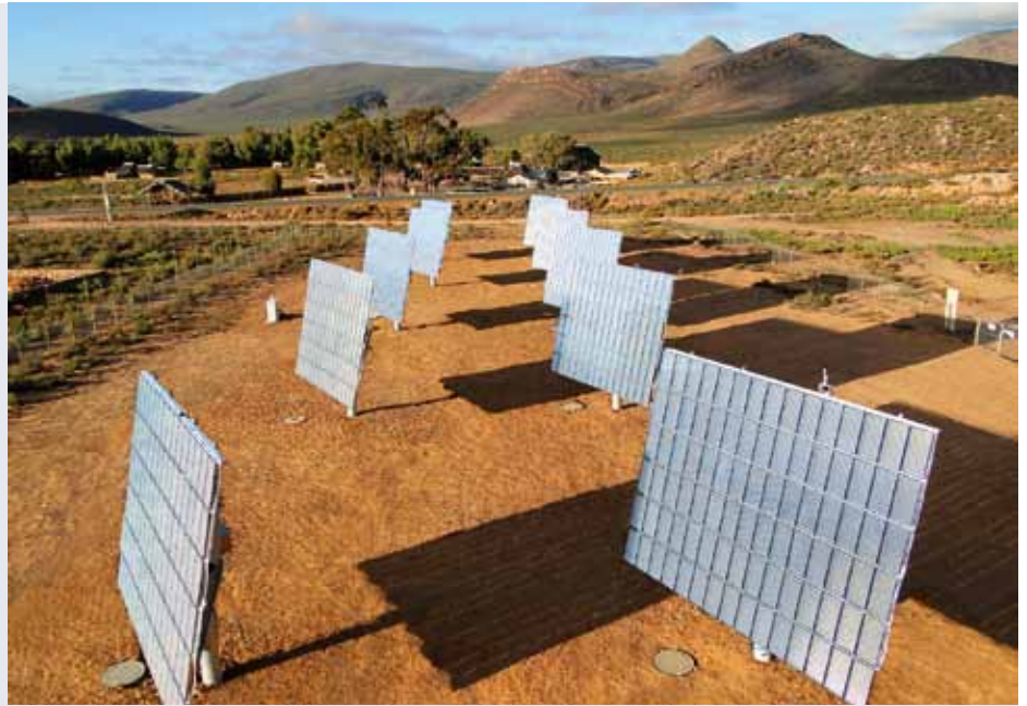
Photovoltaic system in Touwsrivier, near the Aquila Private Game Reserve in South Africa: More than 8,000 trackers facilitate a nominal output of 50 megawatts (MW).
