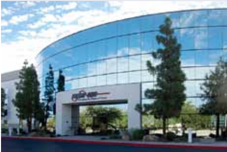
Power-One's 110,000 square foot facility located in Phoenix, AZ
