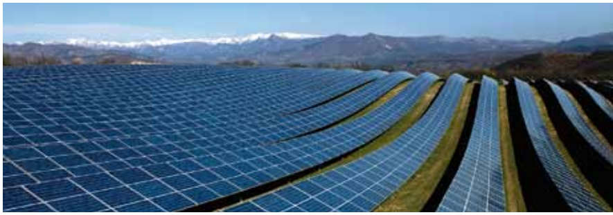
112,000 solar modules with a peak capacity of 31 MWp were installed on a plateau near the French Alps, at the Les Mées solar farm.
