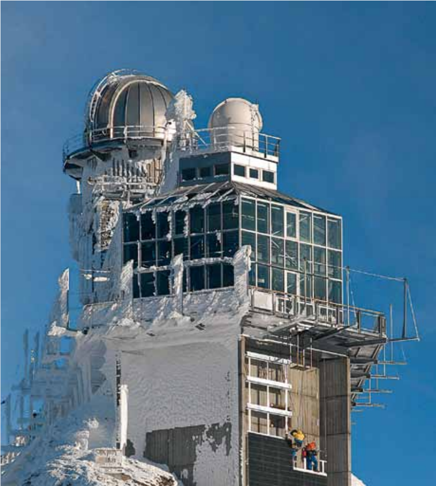
Coping with enormous challenges: The highest grid-connected solar power station in Europe on the Jungfrauoch in Switzerland runs with SolarMax inverters.
