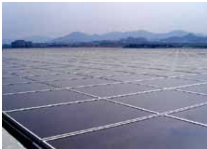
The 1.3 MW PV power plant in Guangming New District, Shenzhen (China) covers about 23,000 square feet of roof space, and is constructed of 13,000 amorphous silicon thin-film modules.
