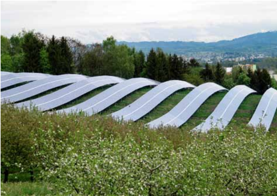
Blended into the landscape: solar power plant in the Czech Republic, 680 kWp
