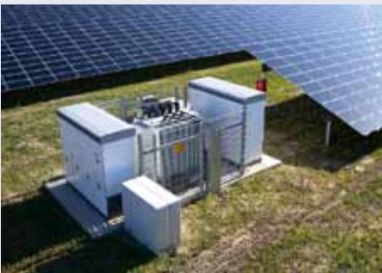
BELECTRIC's Power Conditioning Unit (PCU) combines an intelligent inverter and transformer system with active grid stabilizing technology.
