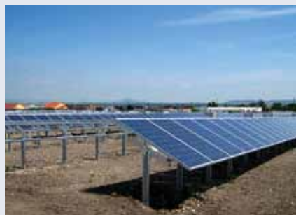
The soil at the location of the 1.48 MW solar power plant near Velký Týnec in the Czech Republic was completely renaturalized when the plant was installed.
