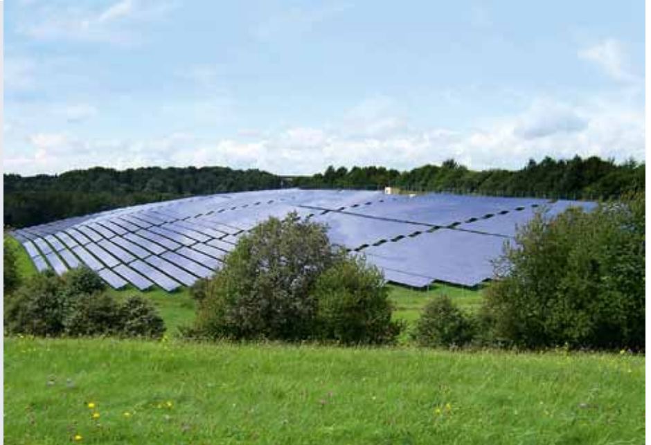
Open field PV power plant, 2.1 MWp, 148 Fronius IG Plus 150 inverters (picture: Eurosol GmbH)
