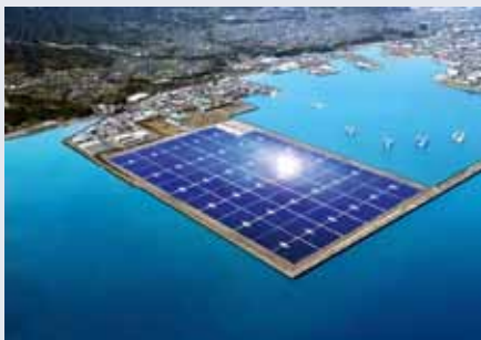
Computer simulation of the solar power station in Kagoshima (Japan). With 70 MW, it is the country's largest photovoltaic power station projected so far.
