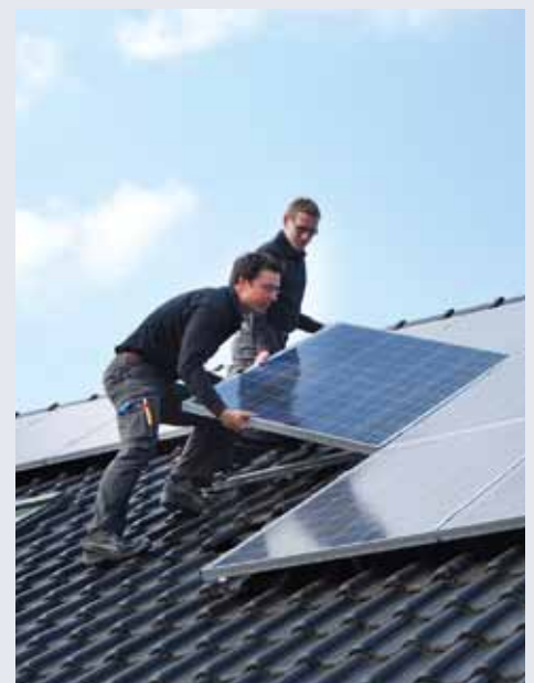
Installation of photovoltaic modules for a roof top plant
