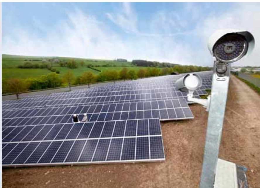
Video monitoring (left) or mechanical locking devices (below) are just two examples for theft protection.
