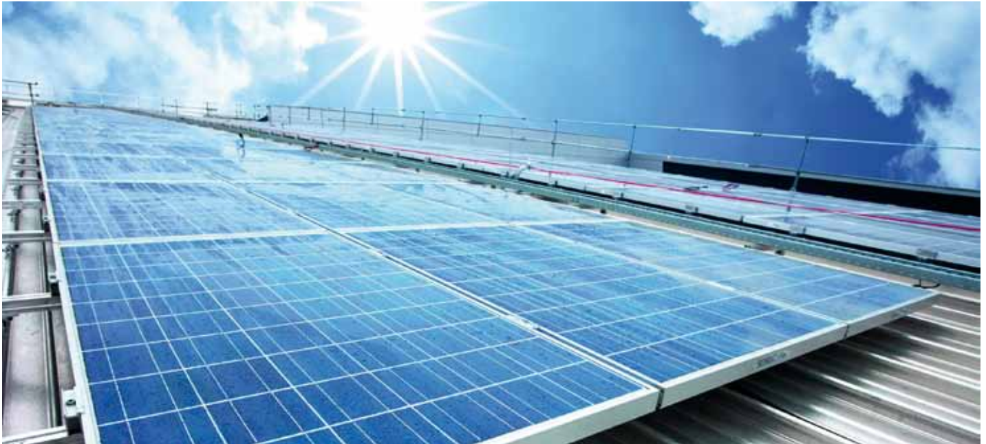
Rhein Main Printing Center in Rüsselsheim, Germany: 2,927 SCHOTT Solar crystalline modules cover 4,771 m 2 of roof surface.
