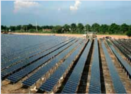
3 MW solar farm in Ayutthaya, 70 kilometers from the Thai capital of Bangkok.
