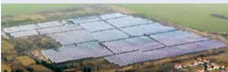
Transparent modules allow architects to build futuristic, façade-integrated PV installations. (top) Masdar PV constructed the largest solar park with thin-film modules in Thuringia (Germany) with a size of 11.7 MWp. (bottom)
