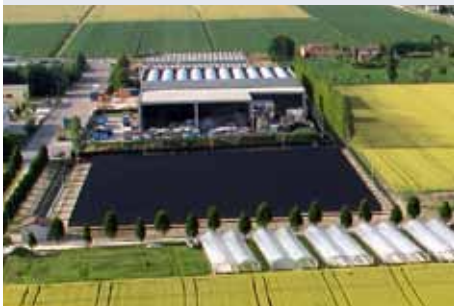
Specifically developed for use in open spaces: PowerMax® SMART modules from AVANCIS (top) Ground mounted system with AVANCIS mod- ules in Italy (bottom)
