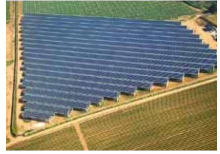
PV-Greenhouses – Food & Energy: combination of an integrated PV system with a standardized greenhouse structure
