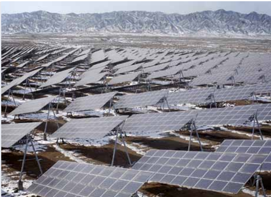
In 2011, China put the Ningxia Tianjingshan PV power plant in Zhongwei into commission. With a capacity of 30 MW, it was the tracking PV power station with the maximum installed capacity in the whole world at the time it was completed.
