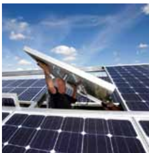
Installing a large-scale photovoltaic plant
