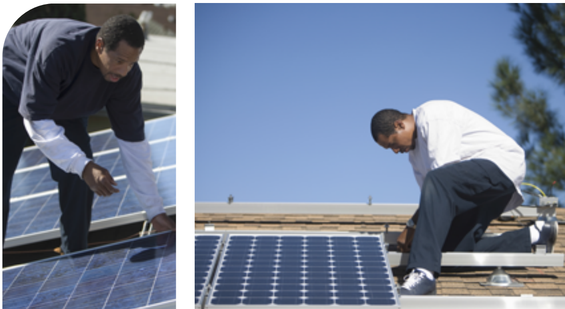
Workers installing solar panels, Shutterstock
