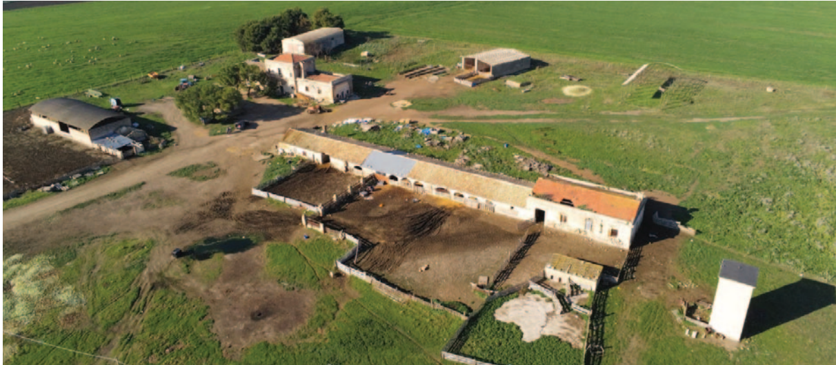
Air view on the ancient farmhouse, which will be restored in the San Severo project.
