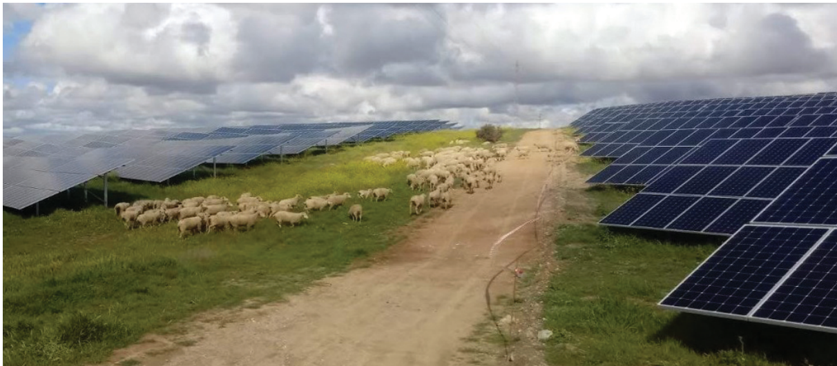
FIGURE 14 IBERDROLA NUÑEZ DE BALBOA PV PLANT
