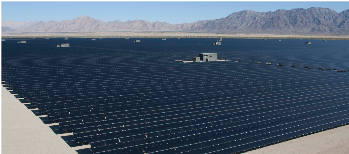
FIGURE 11 TOPAZ SOLAR FARM
