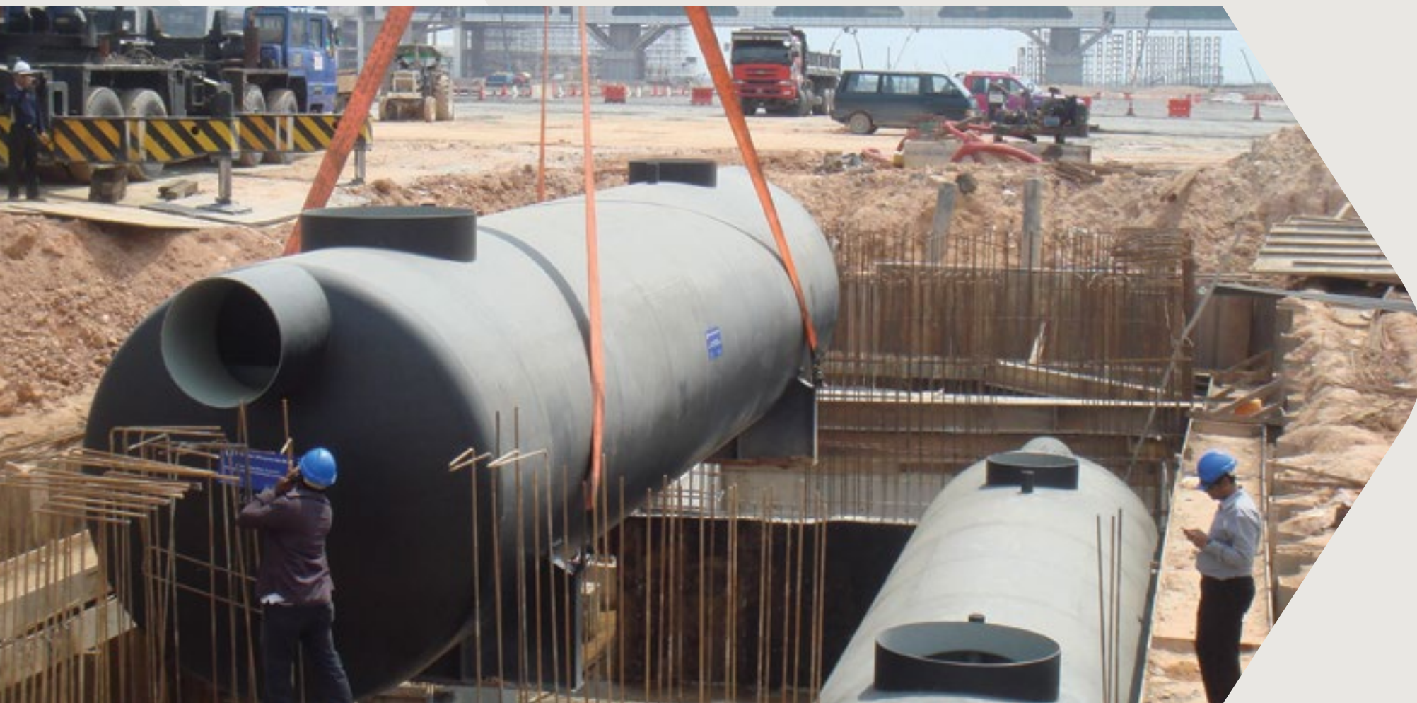
Malaysia Airport Holdings contracted SWA Water Malaysia, a subsidiary of SWA Water Australia, to design, manufacture, install, test and commission an oil separation plant. Image courtesy of SWA Water
